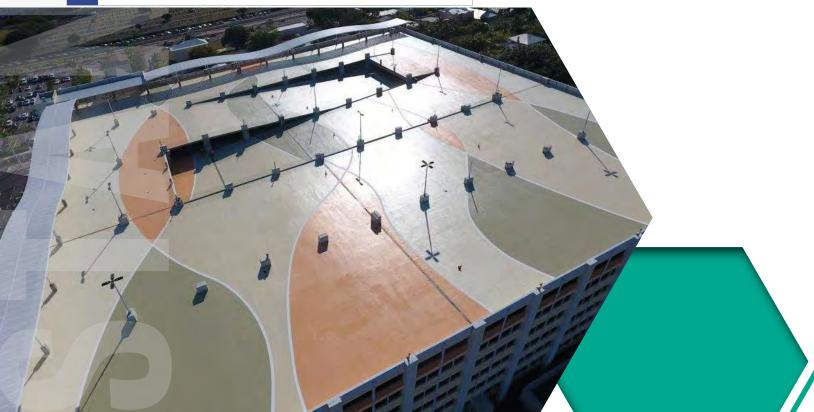
Ideal for waterproofing concrete slabs and protecting occupied areas underneath from water damage while protecting the concrete from the damaging effects of water, deicing salts, chemicals, gasoline, oils and anti-freeze.
